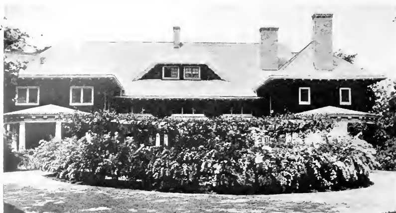
AN INTERESTING EXAMPLE OF MODERN ROOFING IS SHOWN HERE: TRANSITE ASBESTOS SHINGLES, MADE BY THE JOHNS-MANVILLE CO., FORM THE FIREPROOF COVERING.
