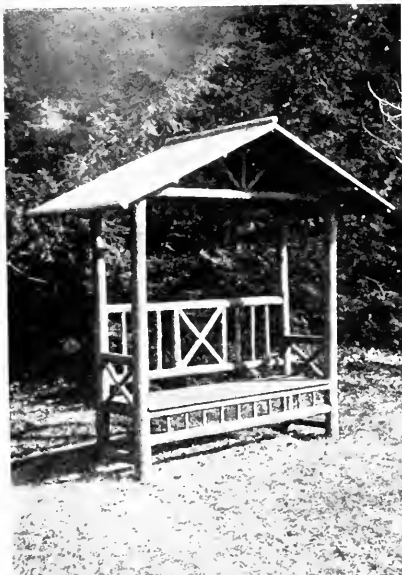
A SEMI-RUSTIC ARBOR WHICH COMPRISES SEAT, SHELTER AND SUPPORT FOR VINES ALL IN ONE STRUCTURE.
