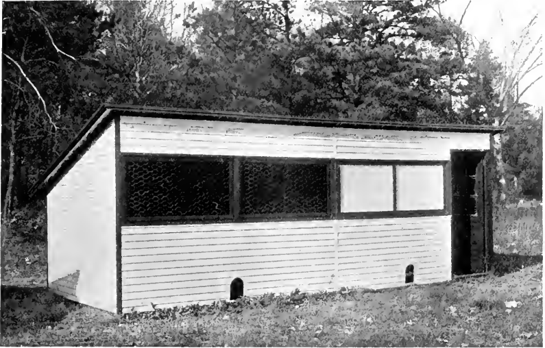
TWO-PEN SECTIONAL POULTRY HOUSE, FITTED WITH DROPPING BOARD, ROOSTS, NESTS, FEED HOPPER, SHELL BOX AND FOUNTAIN: BY PERMISSION OF E. F. HODGSON CO.
