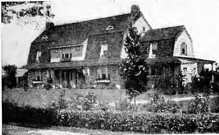
THE WIDE CLAPBOARD WALLS AND SHINGLED GAMBREL ROOFS OF THIS DIGNIFIED, HOSPITABLE-LOOKING HOUSE ARE WELL SUITED TO THE DESIGN: IT IS THE HOME OF HENRY S. ORR AT GARDEN CITY, LONG ISLAND, AND IS AN EXCELLENT INSTANCE OF THE WORK OF AYMAR EMBURY II, WHO HOLDS TO THE BEST COLONIAL AND DUTCH TRADITIONS.
