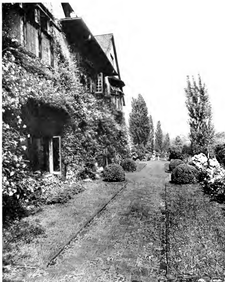
FOUNDATION PLANTING IS ONE OF THE MOST EFFECTIVE MEANS OF PRODUCING HARMONY BETWEEN HOUSE AND GROUNDS: THIS PHOTOGRAPH OF THE HOME OF MRS. JOSEPH BRIGHT AT BRYN MAWR, GIVES A DELIGHTFUL SUGGESTION FOR THE PLANTING OF VINES AND SHRUBS AGAINST THE WALLS: THE GRASS-BORDERED PATHWAY OF BRICK AND THE WELL-PLACED TREES WHICH EMPHASIZE THE GARDEN VISTA ARE ALSO WORTH NOTING.
