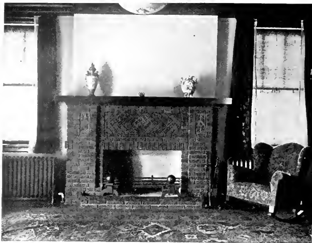
CHIMNEYPiece OF ROUGH-TEXTURED BRICK LAID IN GEOMETRIC DESIGNS: THE WORK OF THE COLONIAL FIREPLACE CO., ONE OF THE CRAFTSMAN EXHIBITORS.
