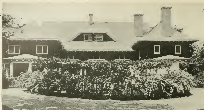
AN INTERESTING EXAMPLE OF MODERN ROOFING IS SHOWN HERE: TRANSITE ASBESTOS SHINGLES, MADE BY THE JOHNS-MANVILLE CO., FORM THE FIREPROOF COVERING.
