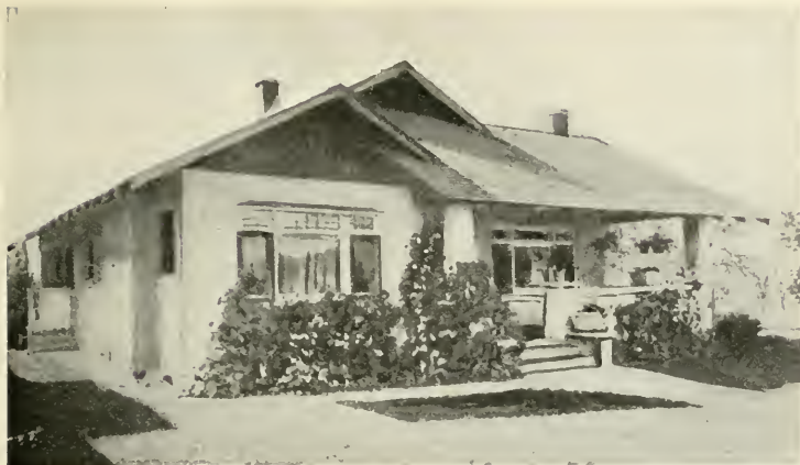
BUNGALOW OF HOLLOW WALL CONCRETE, BUILT BY W. H. RILEY AT RIVERSIDE, CALIFORNIA: A DEMONSTRATION OF THIS TYPE OF CONSTRUCTION, KNOWN AS THE VAN GUILDER SYSTEM, IS AMONG THE INTERESTING FEATURES OF OUR EXPOSITION.
