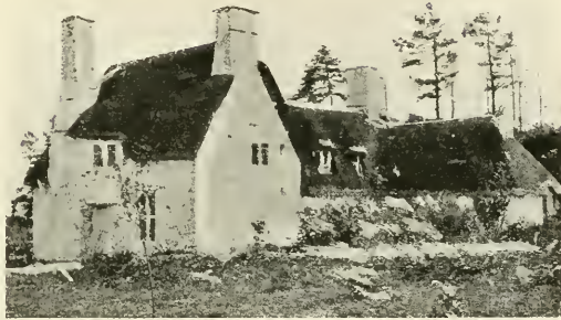
LEA COTTAGE, CHARNWOOD FOREST, LEICESTERSHIRE, ENGLAND; ERNEST GIMSON, ARCHITECT: AN INTERESTING TYPE OF OLD-FASHIONED COUNTRY HOME: PLAN ON PAGE 431.
