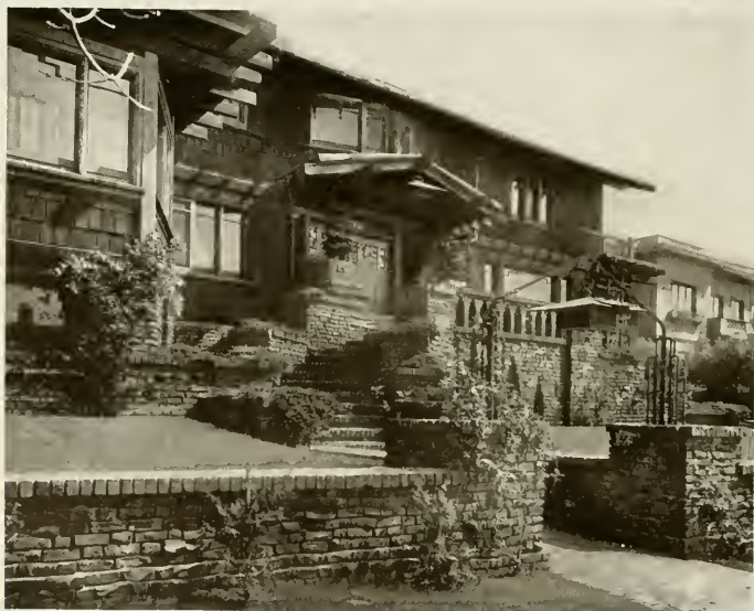
ANOTHER VIEW OF MR. NEILL'S HOME, THE GARDEN WALL OF WHICH IS SHOWN ON PAGE 534: AN INTERESTING EXAMPLE OF BRICK AND COBBLESTONE.
